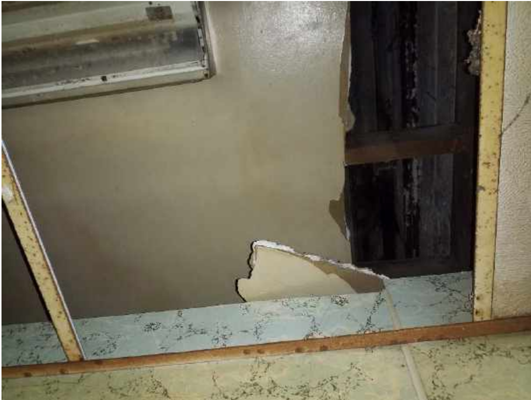
021A, 021 - Gypsum Wallboard System (Wallboard, Joint Tape, and Joint Compound), Room 32, Warehouse offices area
