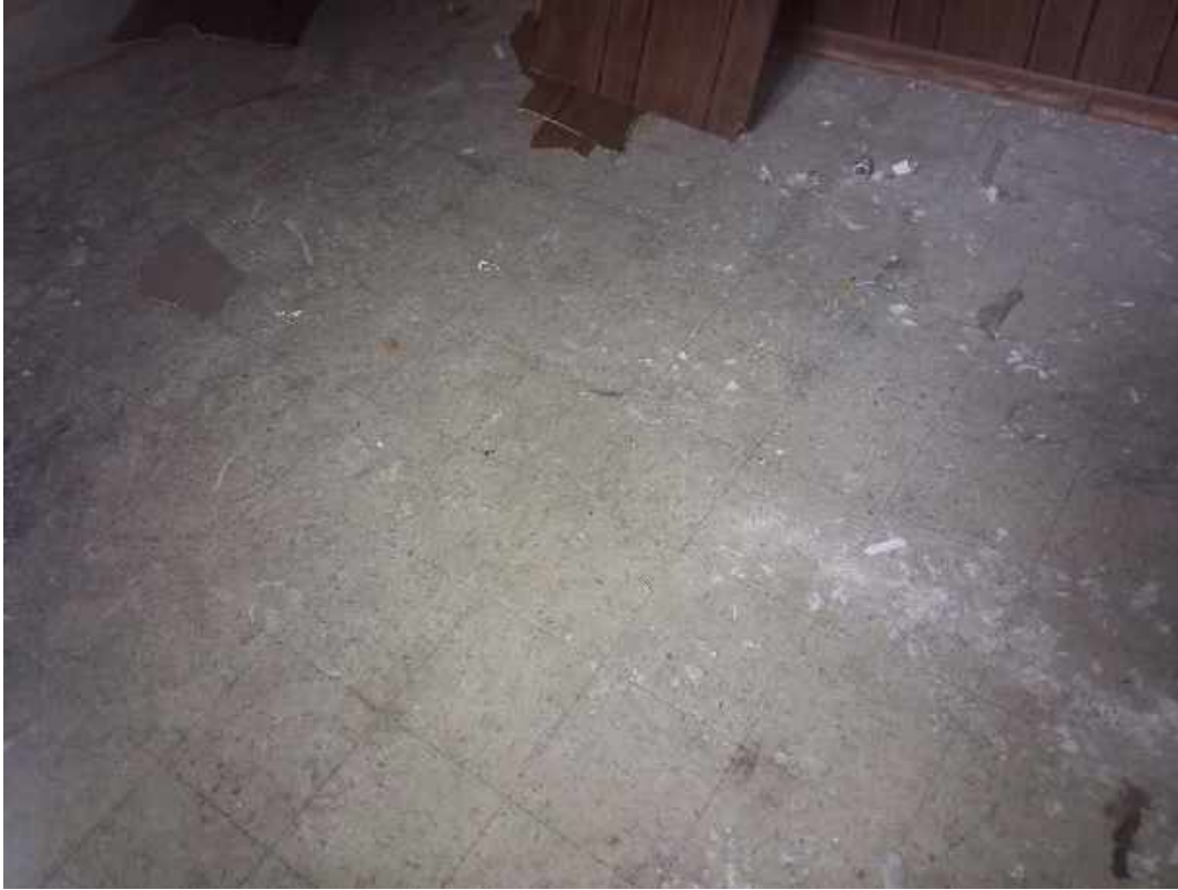
009 - 9"x9" Beige Floor Tile and Mastic, Room 10, 2nd Floor
