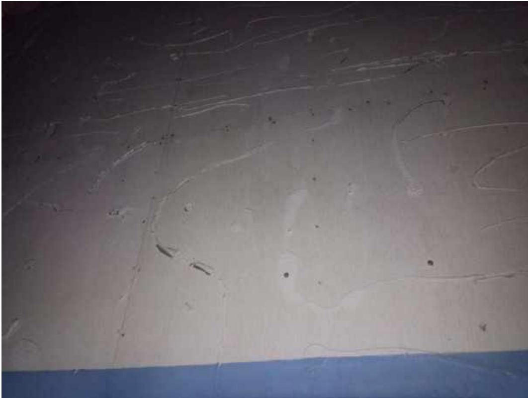
003 - Adhesive on wall, Room 4, 3rd Floor
