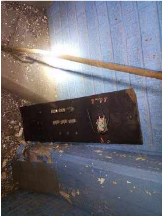
002 - Electrical transite in boxes, Room 17, 2nd Floor
