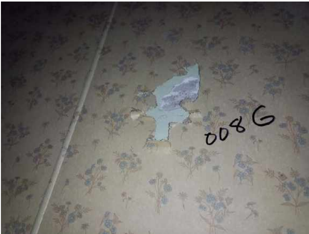
008G, 008 - Hard Plaster , Room 14A, 2nd Floor
