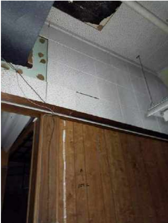
008C Layer 1 White Plaster , 008 - Hard Plaster , Room 14, 2nd Floor This sample is part of a multi-layer sample group
