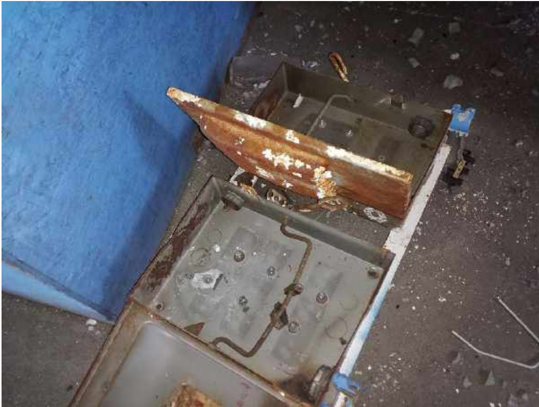
002A, 002 - Electrical transite in boxes, Room 9, 3rd Floor
