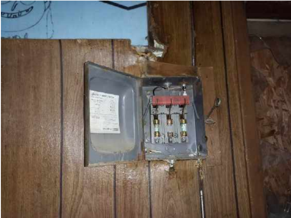
002 - Electrical transite in boxes, Room 39, Warehouse offices area
