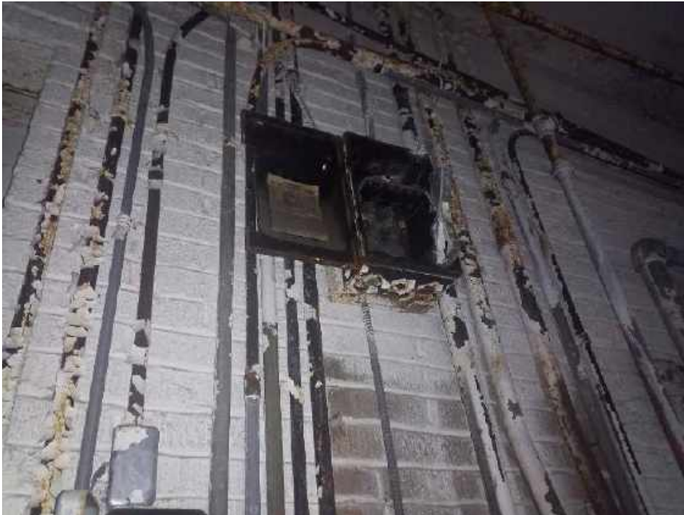
002 - Electrical transite in boxes, Room 3, 3rd Floor
