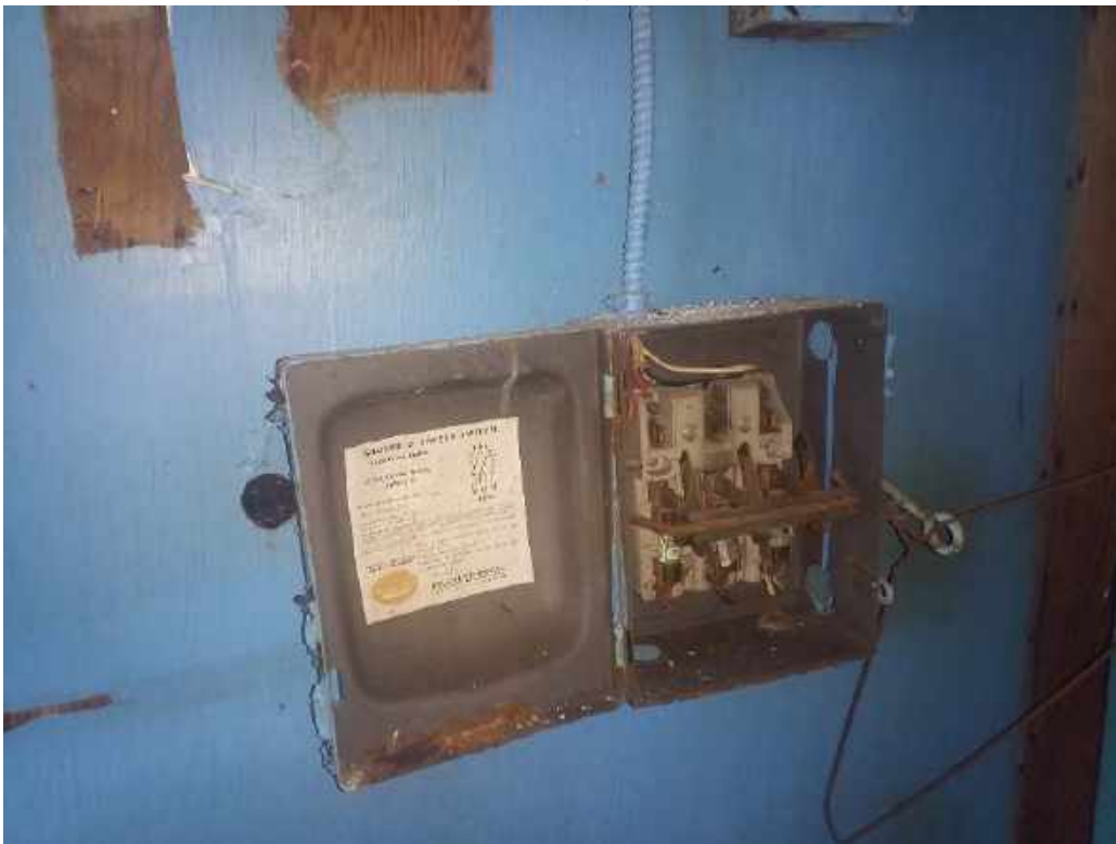
002 - Electrical transite in boxes, Room 5, 3rd Floor
