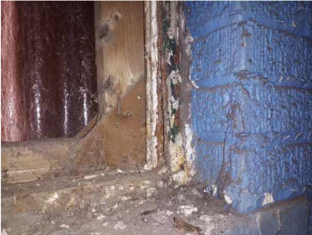
004A, 004 - Caulk, Window, Room 27, 1st floor under offices
