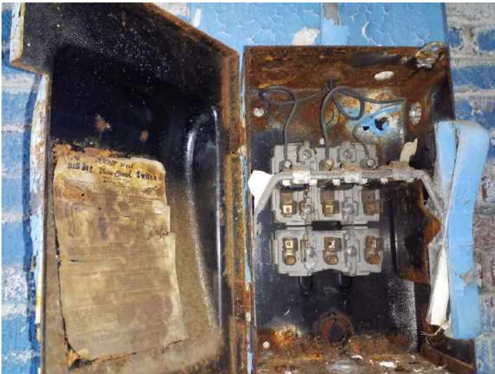
002B, 002 - Electrical transite in boxes, Room 9, 3rd Floor
