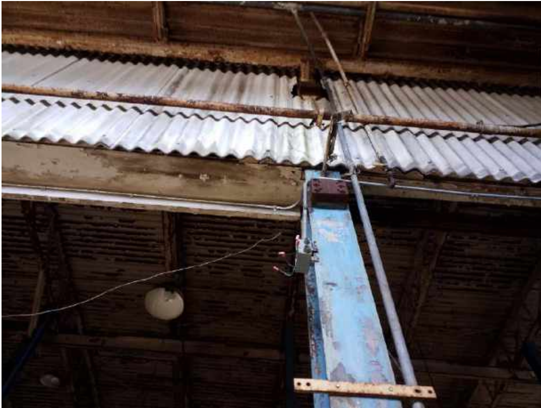
025A, 025 - corrugated transite, Room 44, Large L shaped warehouse
