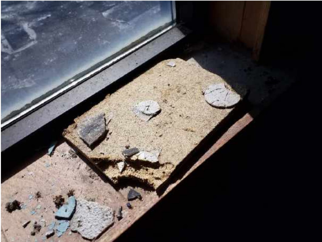
017A, 017 - Black Ceiling tile mastic, Room 15, 2nd Floor
