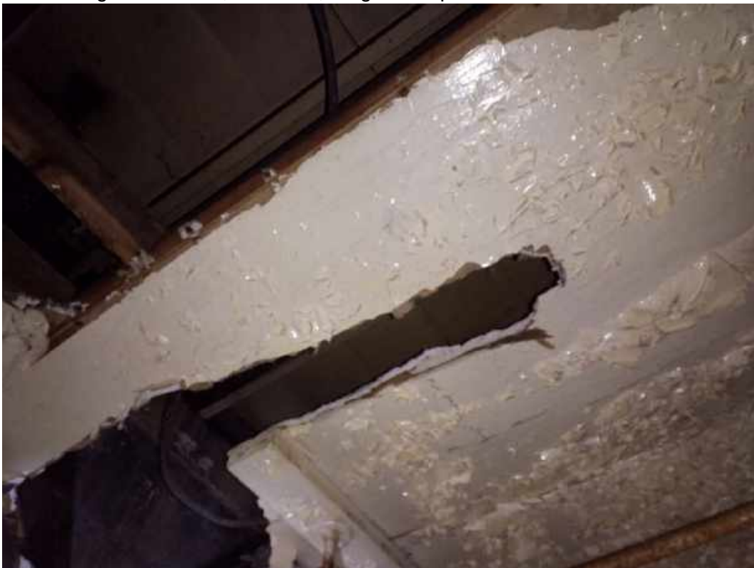
025 - corrugated transite, Room 44, Large L shaped warehouse
