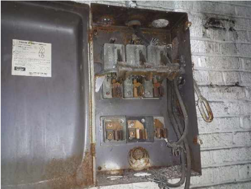
002 - Electrical transite in boxes, Garage next to Room 24 by mens restroom, 1st floor under offices
