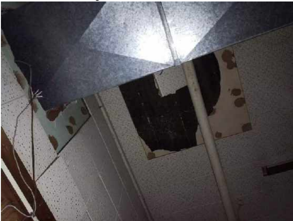
017B, 017 - Black Ceiling tile mastic, Room 14, 2nd Floor
