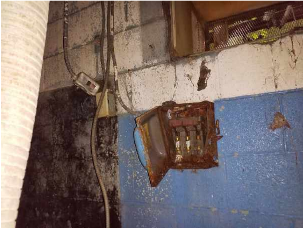
002 - Electrical transite in boxes, Room 41, Large L shaped warehouse
