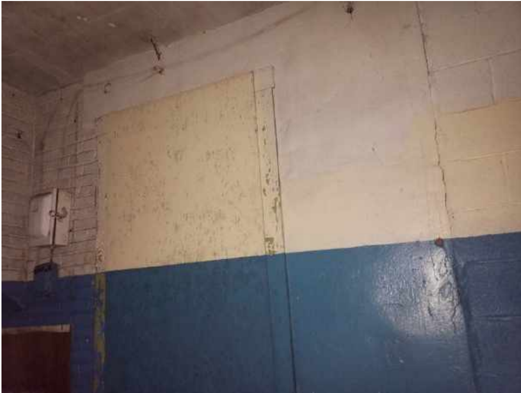
008A, 008 - Hard Plaster , Room 27, 1st floor under offices
