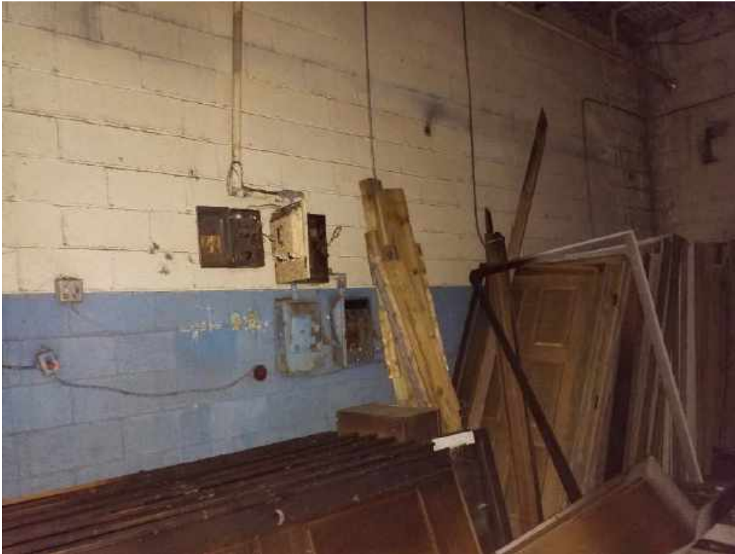
002 - Electrical transite in boxes, Room 45, Large L shaped warehouse
