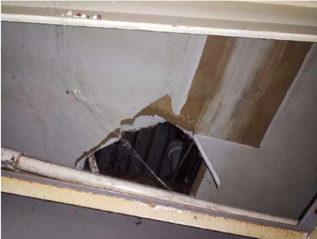
021B, 021 - Gypsum Wallboard System (Wallboard, Joint Tape, and Joint Compound), Room 33, Warehouse offices area
