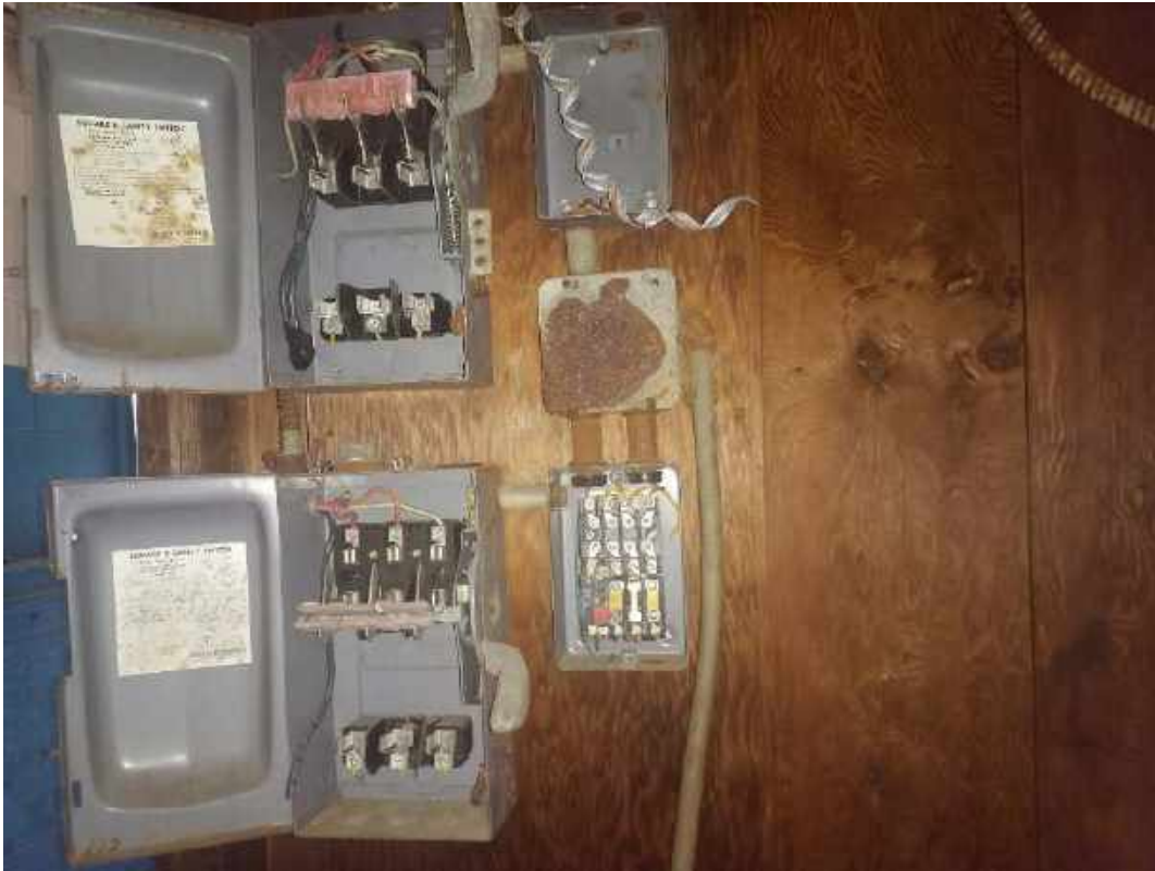
002 - Electrical transite in boxes, Room 2, 3rd Floor
