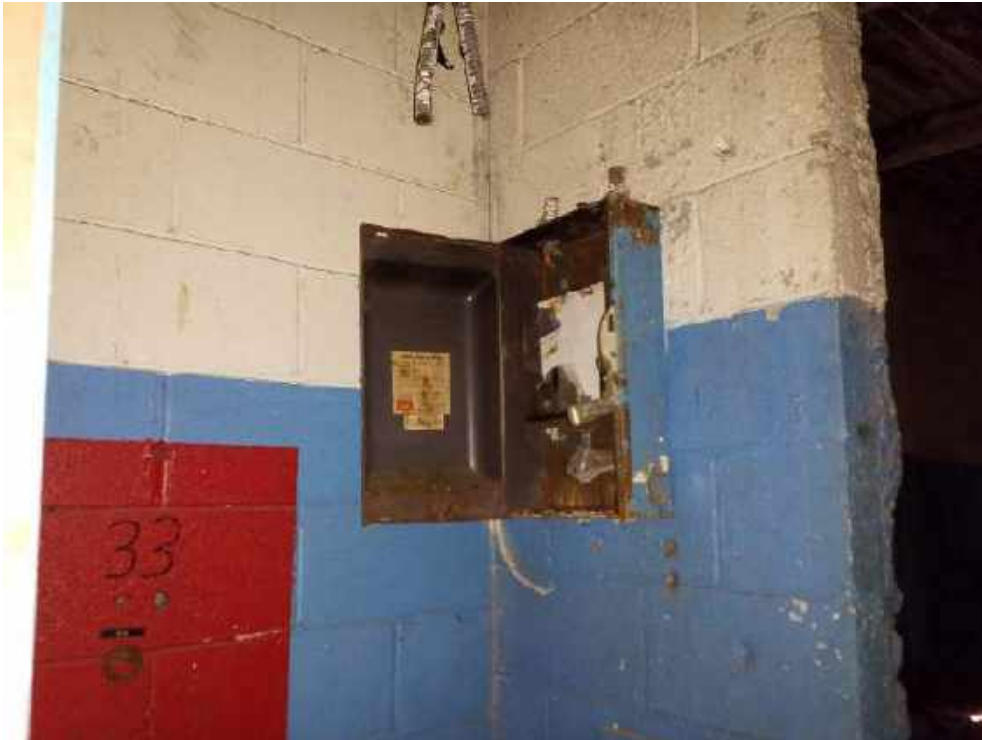
002 - Electrical transite in boxes, Room 31, Warehouse offices area
