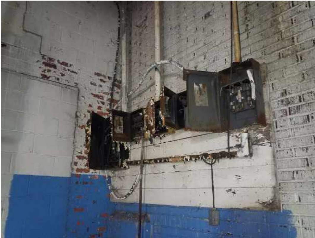
002 - Electrical transite in boxes, Room 28, North 1st Floor
