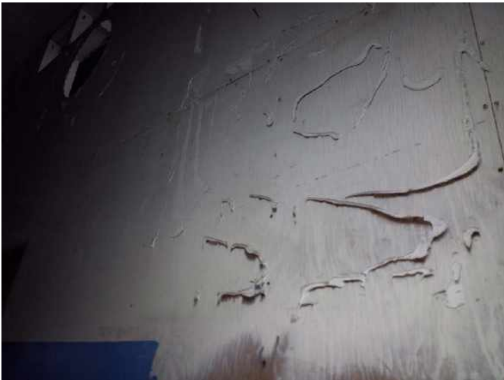
003B, 003 - Adhesive on wall, Room 4, 3rd Floor
