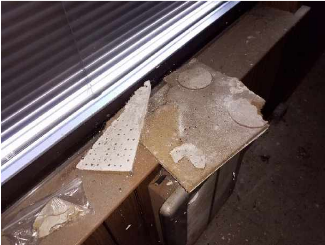
007A, 007 - Brown Ceiling tile mastic, Room 10, 2nd Floor
