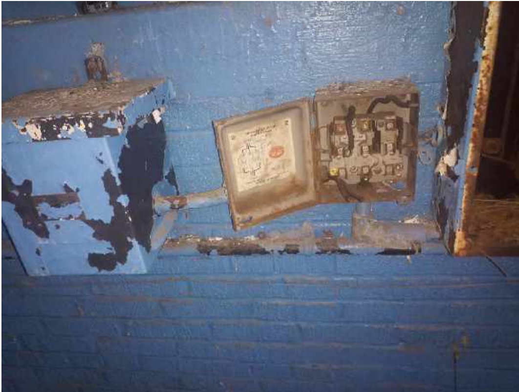
002 - Electrical transite in boxes, Room 3, 3rd Floor
