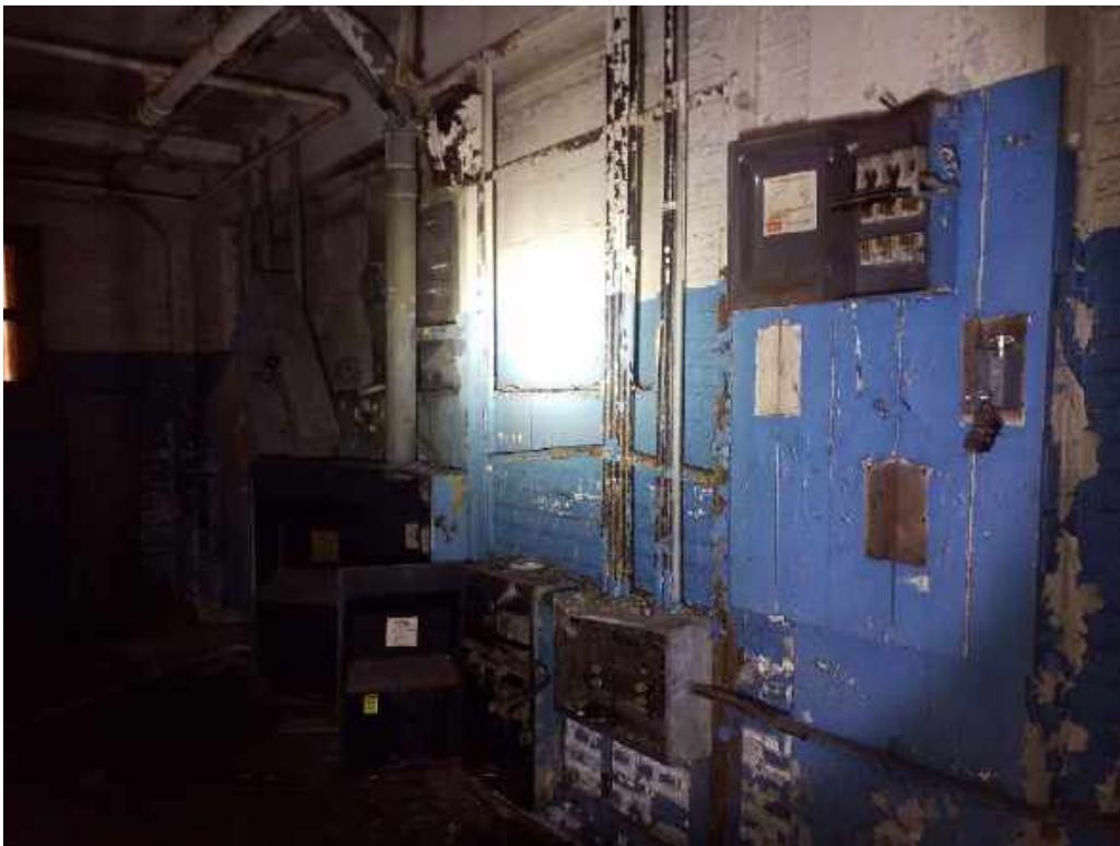
002 - Electrical transite in boxes, Room 27, 1st floor under offices
