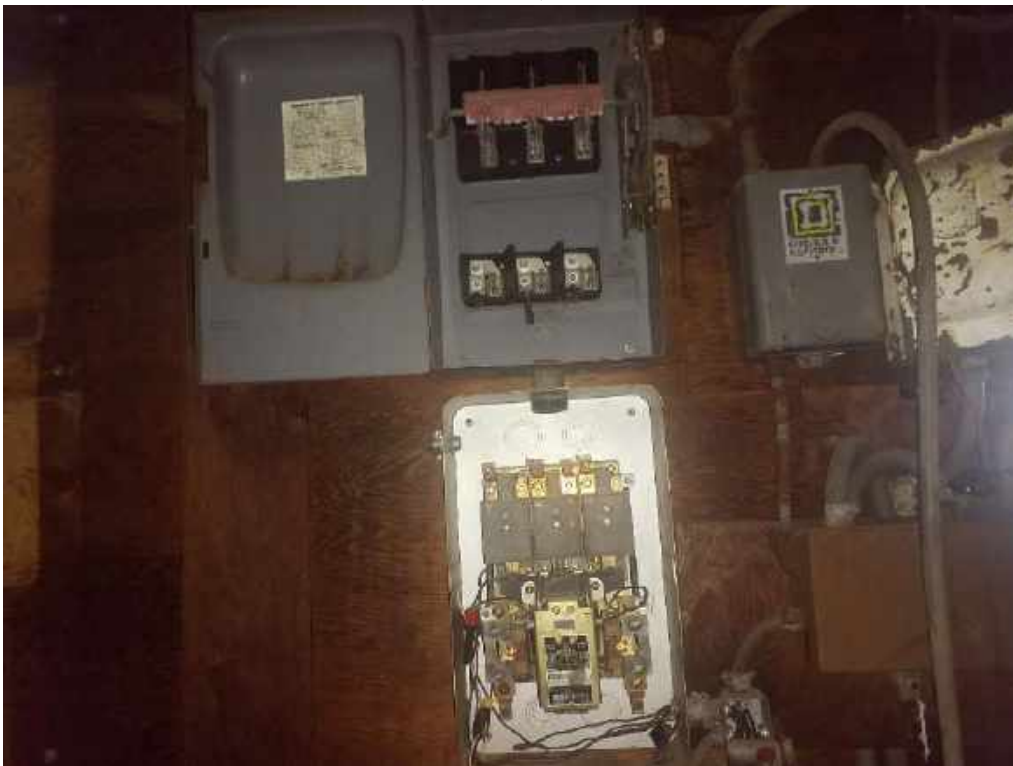
002 - Electrical transite in boxes, Room 2, 3rd Floor
