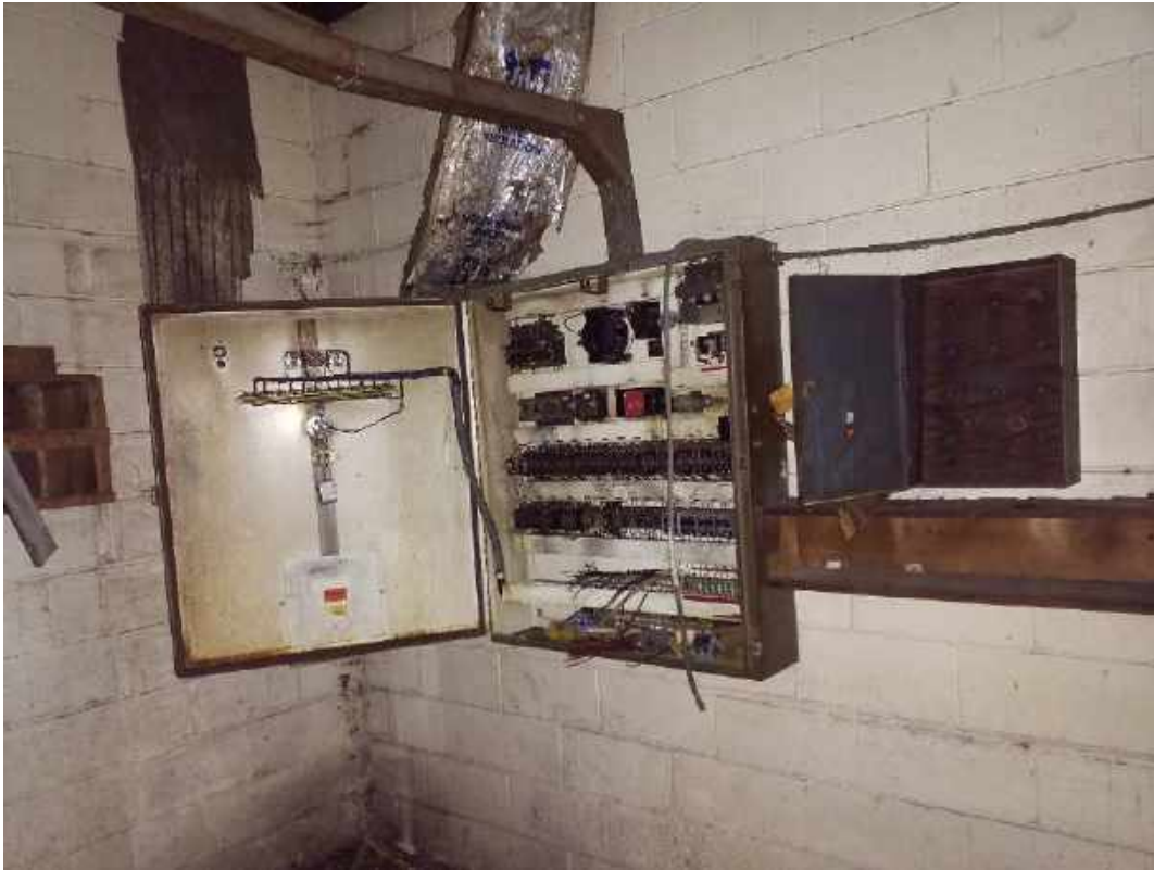
002 - Electrical transite in boxes, Room 47, Back warehouse and lean-to
