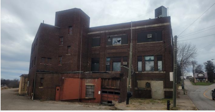
South Side of Bldg
