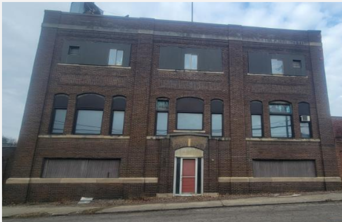
S. Main Street (East Side of Bldg)
